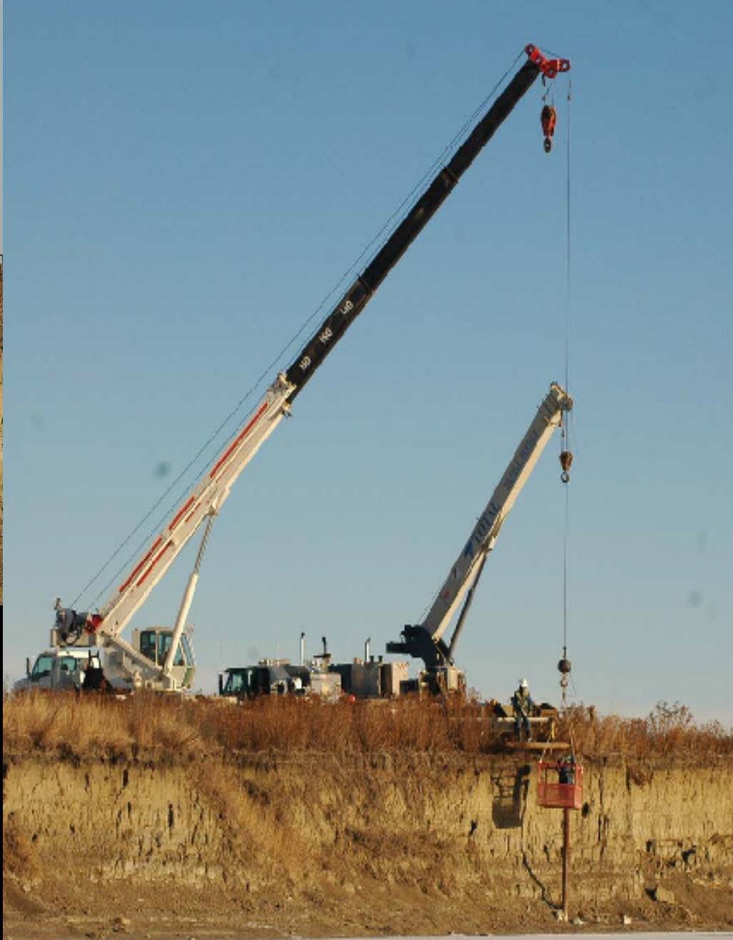
Camerina Petroleum 00/10-09-061-27W4/0 Removing Casing Stub in Pembina River
