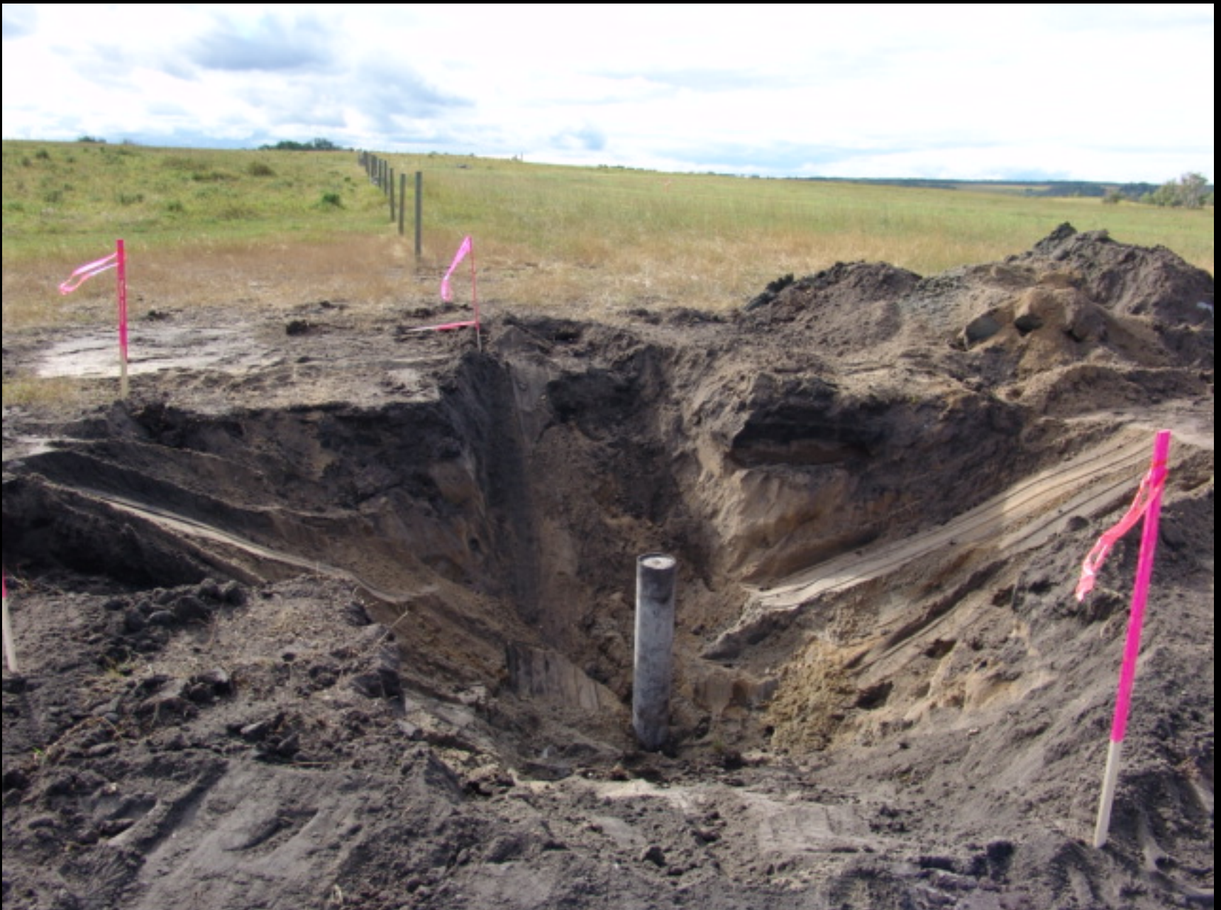
55-02W4 Casing Stub Exposed
